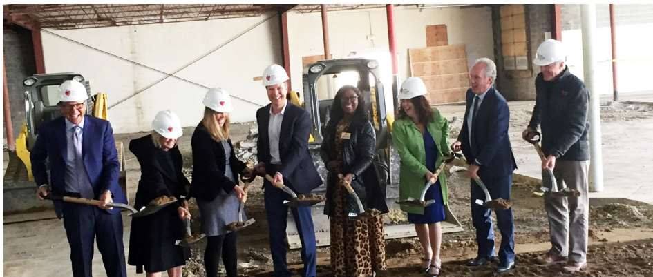
Staff and board members from Dare to Care, Yum! Brands and Catholic Charities joined Mayor Greg Fischer to break ground on the Dare to Care Community Kitchen.
